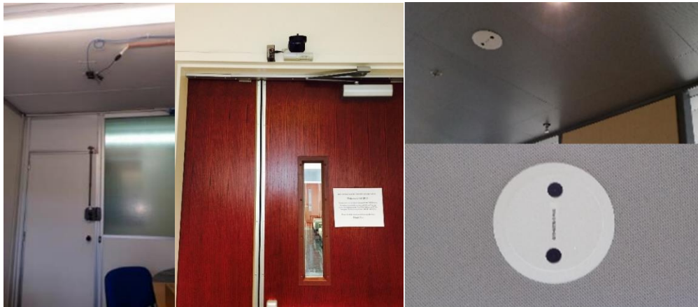
a) Micro camera through RaspberryPi at University of Calabria (Italy) (Picture by Dafni Mora)
